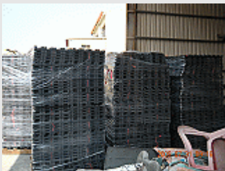
recycle from job site
