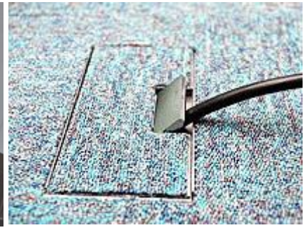
Steel lid topped by carpet tile
