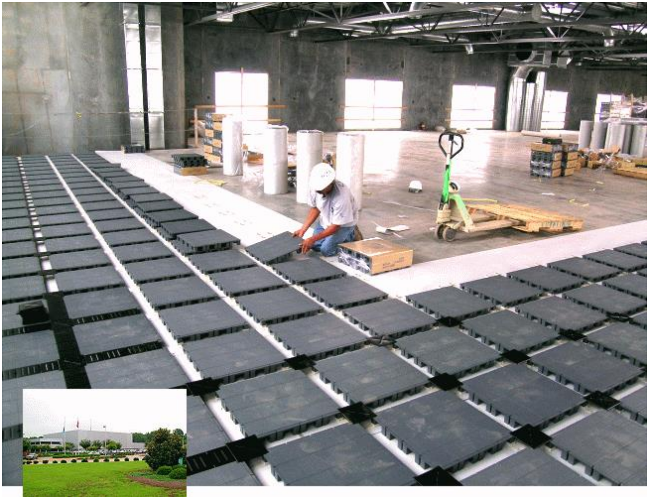
a multi-nation company factory office, USA
